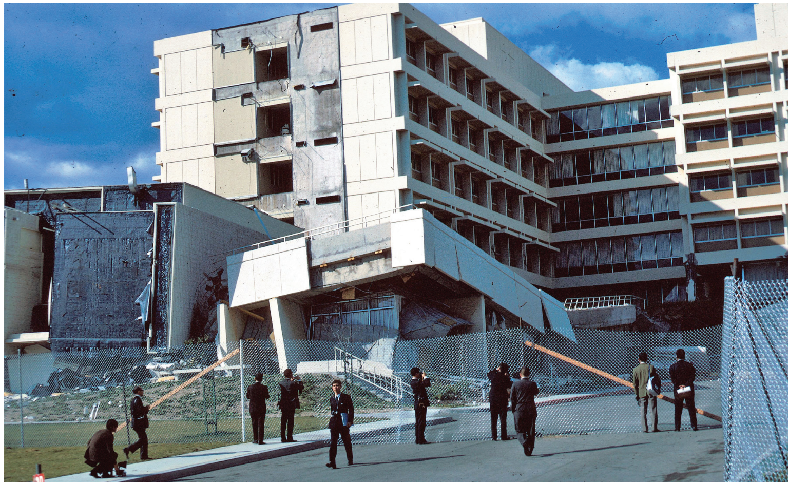
This fallen stair tower at a hospital was the result of the San Fernando Earthquake of Feb. 9, 1971. (© U.S. Geological Survey)
