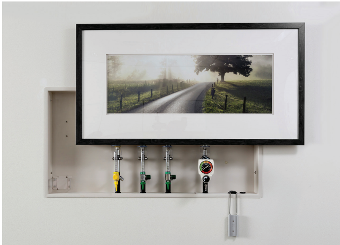
Access to medical gas outlets can be concealed behind artwork in hospitals when not needed. (Photo © Modular Services)
